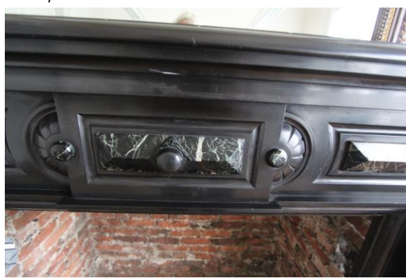
Detailering schouw in leefkamer H1-2
