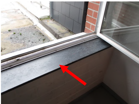
ZM/1: Venstertabletten in asbestcement
