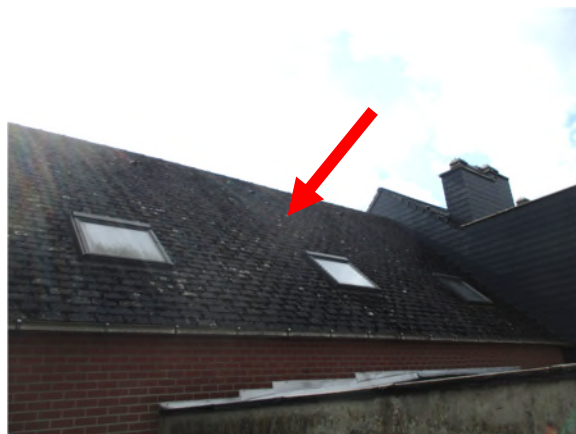
LRK17/1: Dakleien in asbestcement
