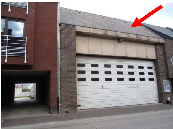
LRK17/1: Dakleien in asbestcement
