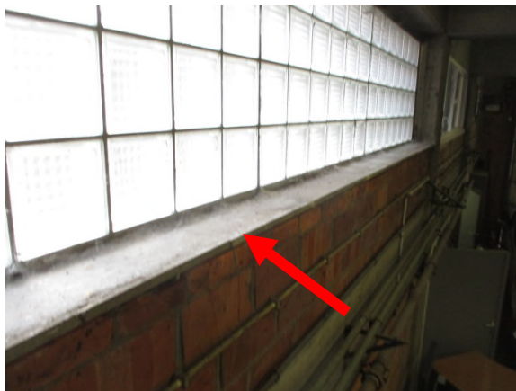
ZM/1: Venstertabletten in asbestcement
